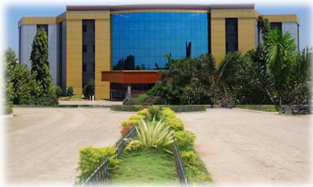
Fig.1: PSVP Engineering College, Ponmar, Chennai - 600127
